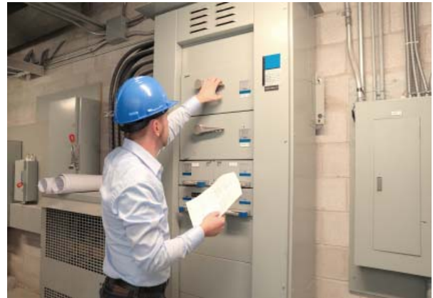
The right building services increase efficiency
